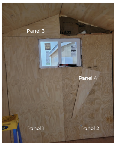
Photo: Wall #2 in Process
