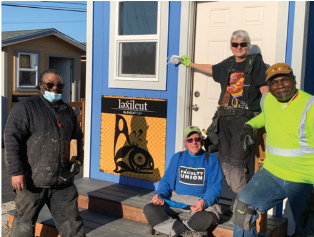
LIHI Construction Crew: (Pictured from left) Abdul Jones, Guy Astley, Stephanie Colbert, James Raye
