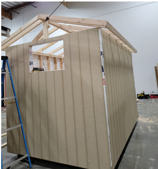
Photo: Roof Frames Attached
