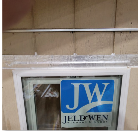
Photo: Window Top Membrane Flashing
