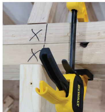
Photo: Roof Ridge Beams
