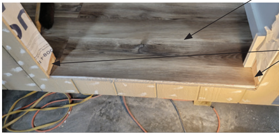
Photo: Cut-out Doorway Plate
