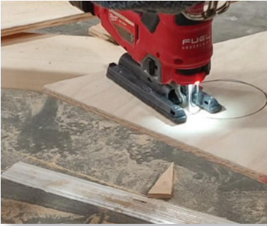
Photo: Cutting Vent Hole
