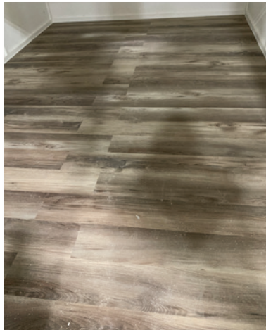
Photo: Flooring Completed
