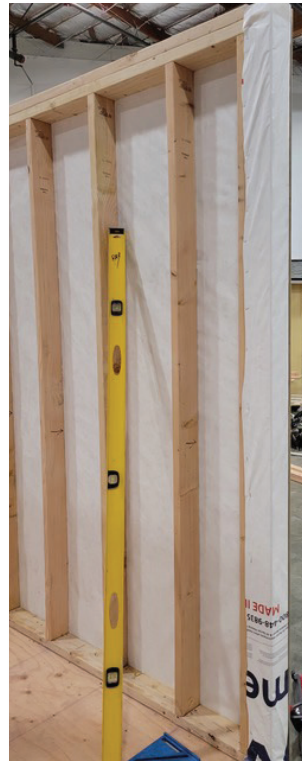
Photo: Wrap Around Corner of wall
