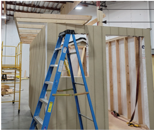
Photo: Raising Roof Frame Set Up
