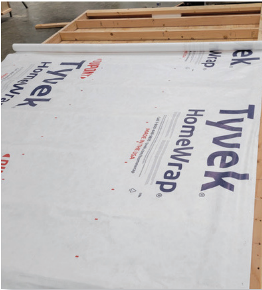
Photo: Installing House Wrap
