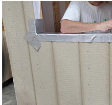
Photo: Window Sill Flashing Installed
