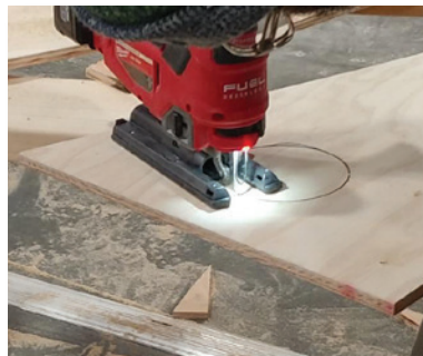
Photo: Cutting Vent Hole
