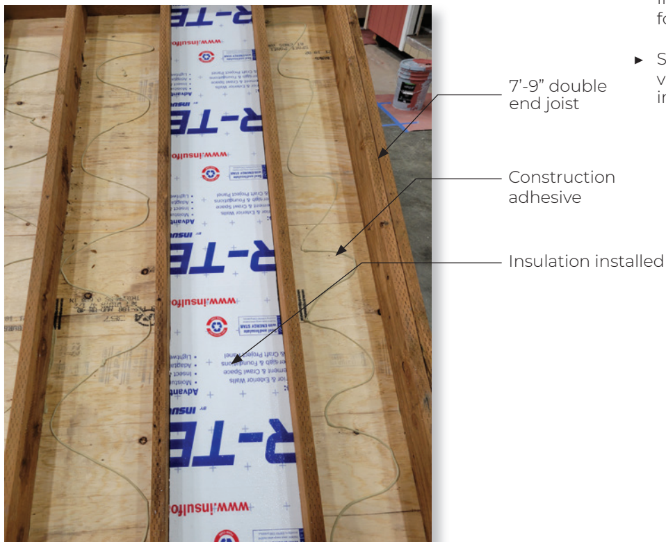
Photo: Installing Rigid Insulation Floor
