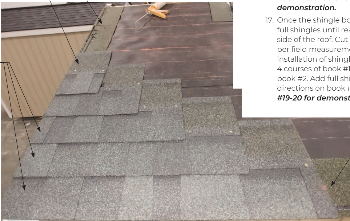
Photo: First Shingle Book Installed
