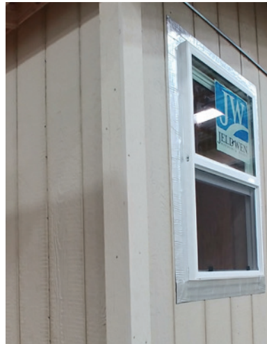
Photo: Exterior Corner Trim Boards
