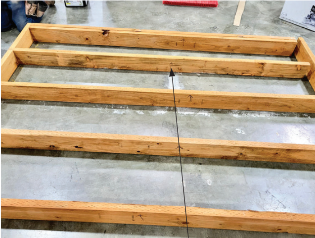
Photo: Floor Joist Layout
