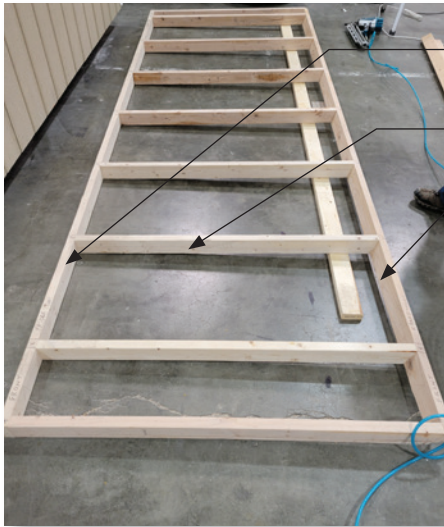
Photo: Roof Framing on Ground
