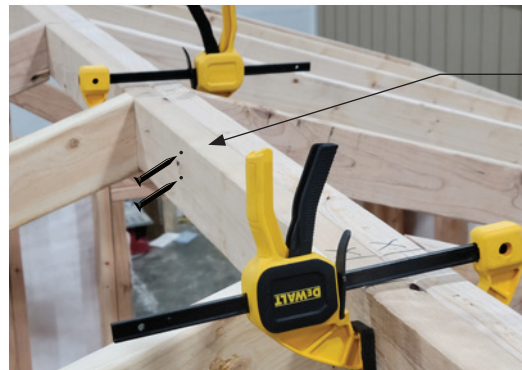
Photo: Ridge Beams Clamped
