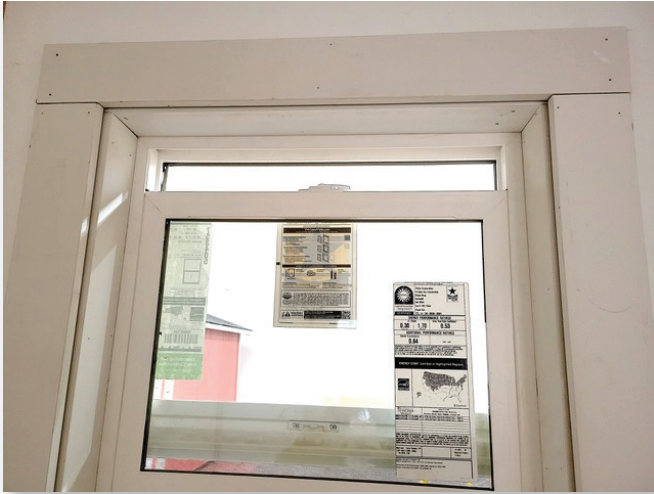
Photo: Window Head & Side Trim
