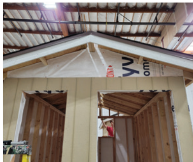
Photo: Wrap Installed
