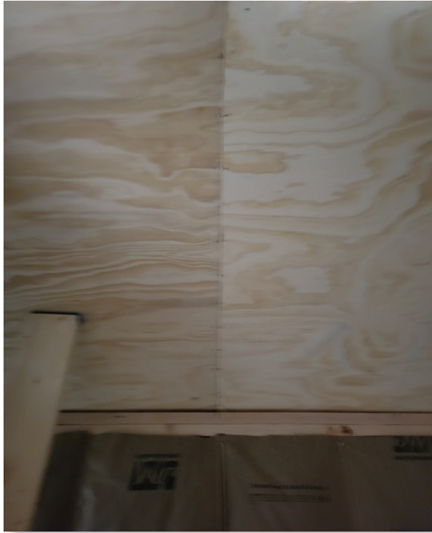
Photo: Ceiling Panels Joined
