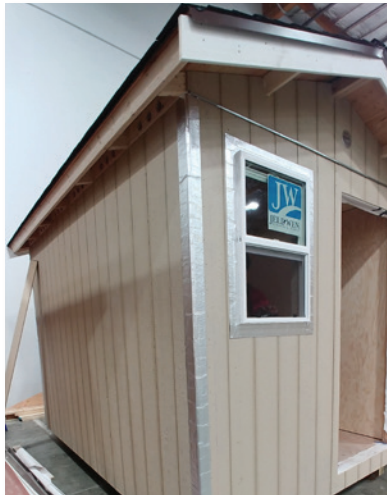
Photo: Flashing Exterior Corners B4 Trim
