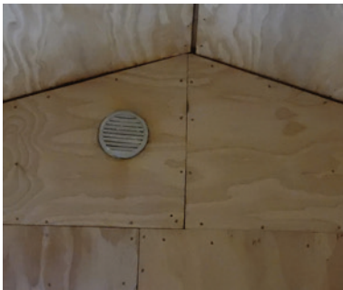
Photo: Louvered Vent on Wall #3 Interior
