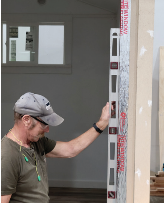
Photo: Checking with Level on Door Frame
