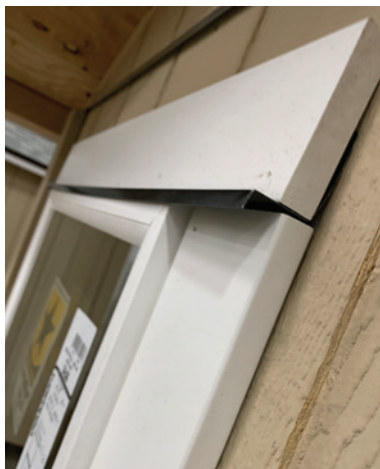
Photo: Window Z-flashing Detail
