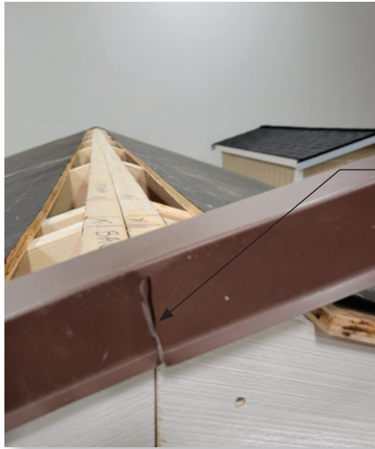
Photo: Drip Edge Flashing Ridge Cut
