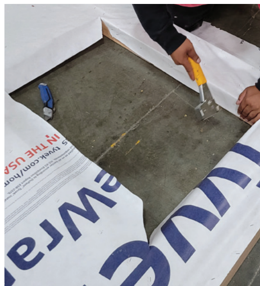
Photo: Installing Wrap Around Window Opening
