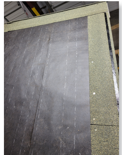
Photo: Starter Strips Installed
