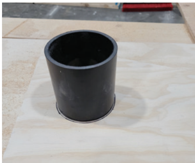
Photo: Tracing Vent Circle on Plywood
