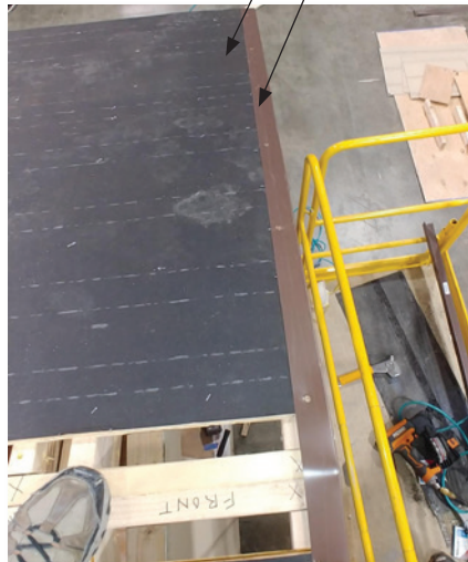
Photo: Drip Edge Flashing Finished
