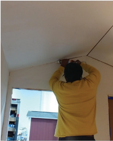
Photo: Caulking the Interior
