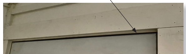
Photo: Door Trim Reveal
