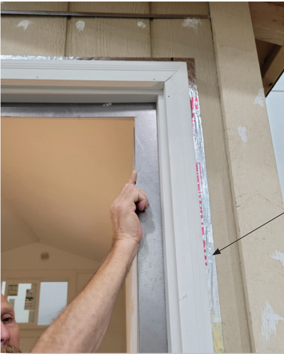
Photo: Checking Door for Square
