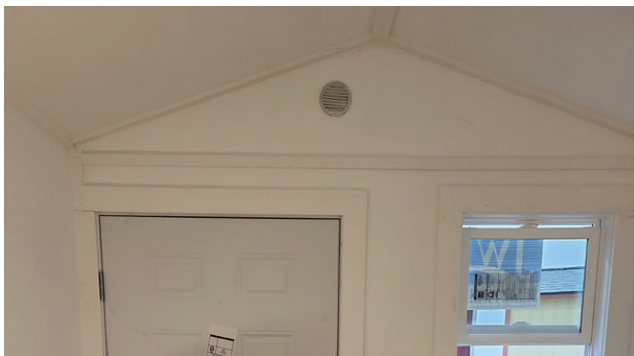
Photo: Front Wall Trim Complete
