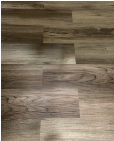
Photo: Finished Flooring Pattern
