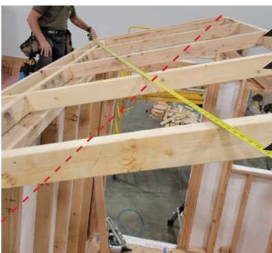
Photo: Checking Diagonals on Roof Frame
