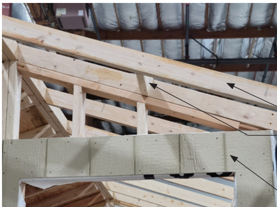
Photo: Rake Rafter Blocking
