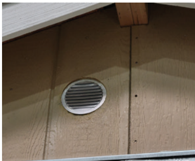
Photo: Louvered Vent on Wall #2 Exterior
