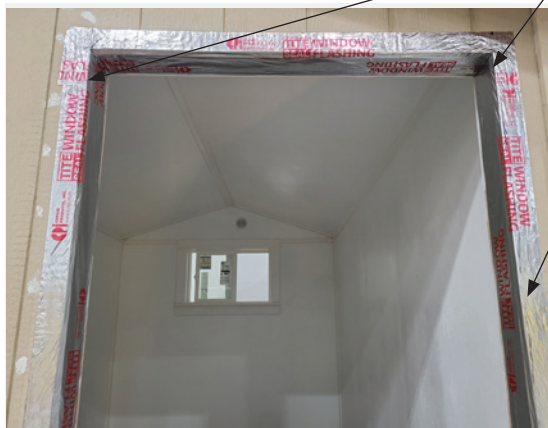
Photo: Door Flashing
