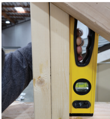
Photo: Level on Roof Ridge Posts
