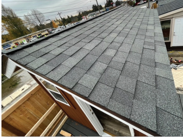
Photo: Roofing Complete One Side
