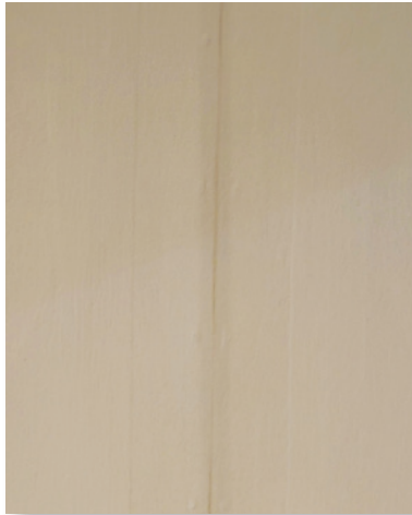
Photo: Seam Tape Applied with Primer
