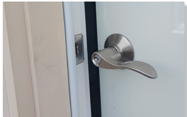
Photo: Completed Lockset Installation
