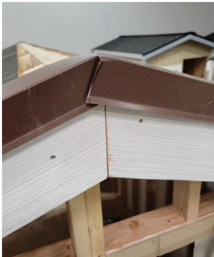
Photo: Drip Edge Flashing Bend
