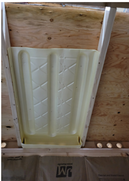
Photo: Completed Baffle Installation
