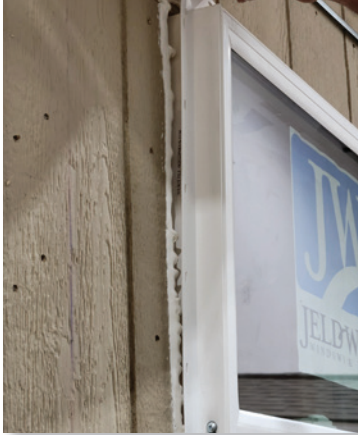
Photo: Caulking Behind Window Installation
