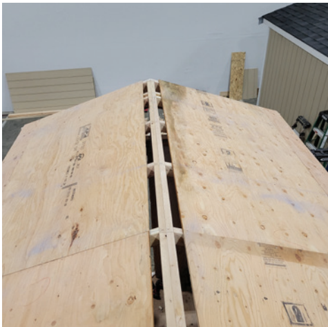
Photo: Ridge Air Gap
