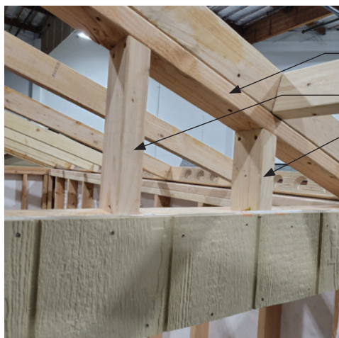
Photo: Gable Wall Upper Triangle
