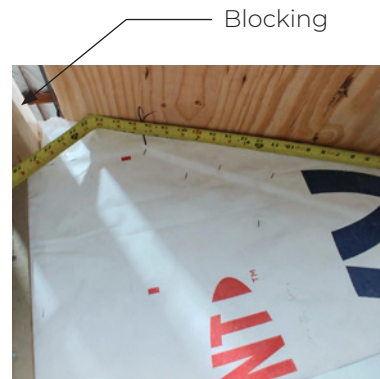
Photo: Measuring for Blocking Cut-out
