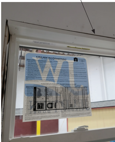
Photo: Window Casing Top Piece
