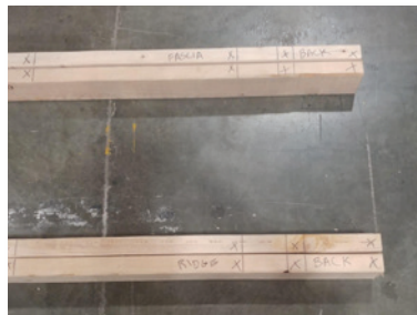
Photo: Rafter Layout on Fascia and Ridge Beam
