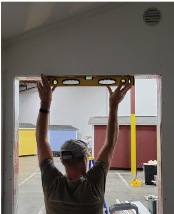
Photo: Checking with Level on Door Frame Top
