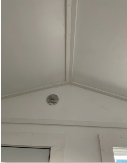
Photo: Interior Ceiling Trim Front Wall
