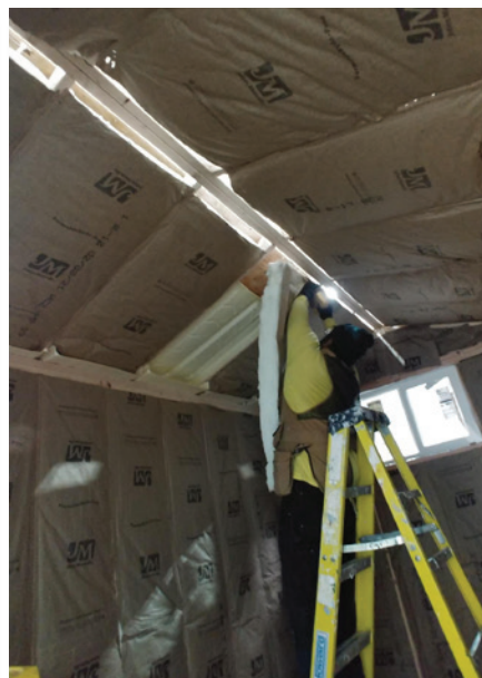
Photo: Ceiling Batt Insulation
