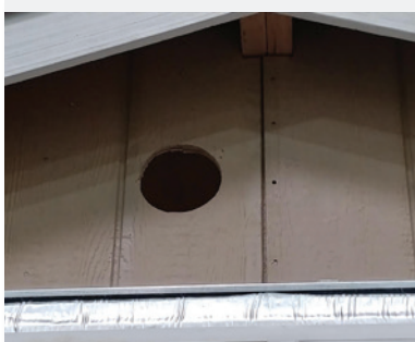
Photo: Wall #2 Upper Sheathing with Vent Hole
