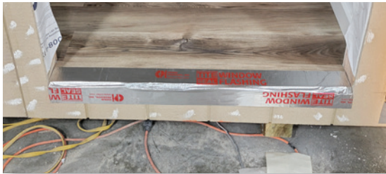
Photo: Door Lower Flashing
