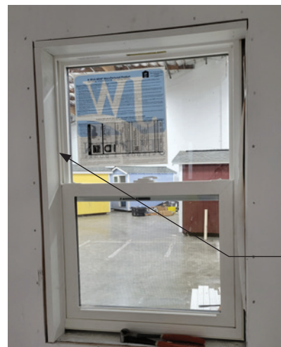
Photo: Window Casing Side Pieces
