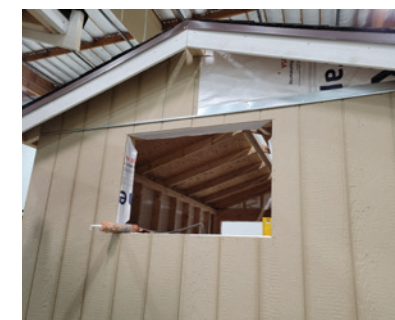
Photo: Left Side Sheathing Installed
