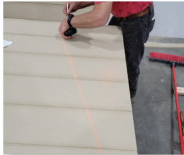
Photo: Pattern Layout on Sheathing
