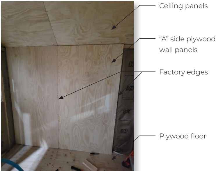
Photo: Interior Panels 1 & 2 Installed
