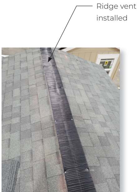
Photo: Ridge Vent Installation
