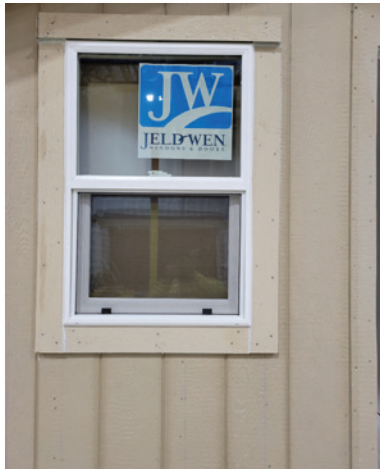
Photo: Wall #3 Window Exterior Trim
