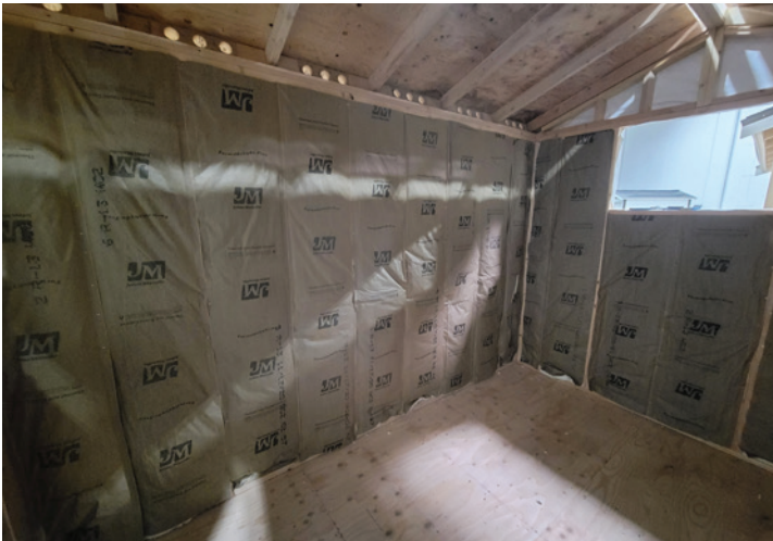
Photo: Wall Batt Insulation
