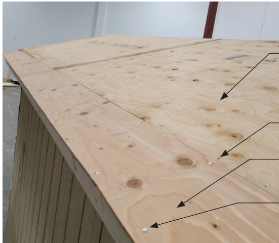
Photo: Roof Sheathing & Nailing
