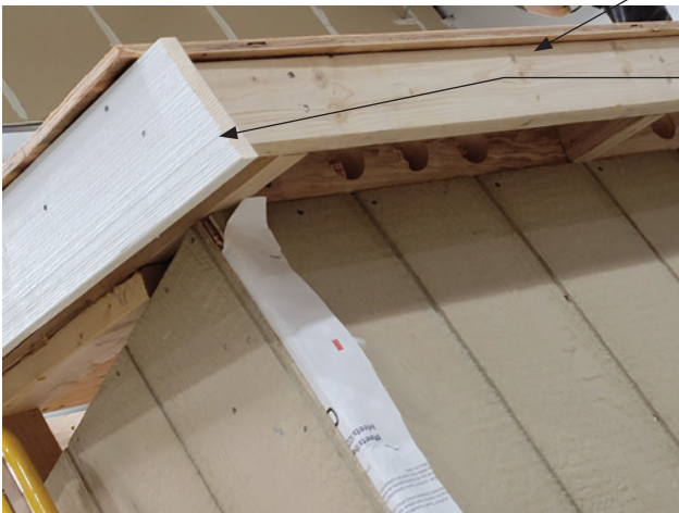
Photo: Barge Trim Overhang
