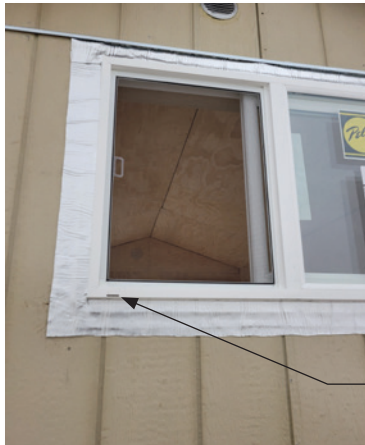
Photo: Window Membrane Flashing Complete
