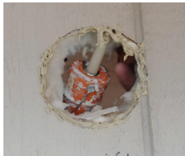
Photo: Caulking Vent Hole
