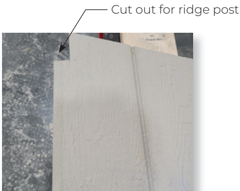
Photo: Ridge Post Cut-out
