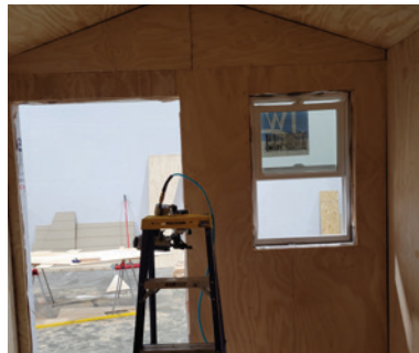
Photo: Wall #3 Interior Covering Completed
