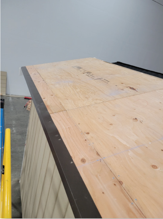
Photo: Eave Flashing
