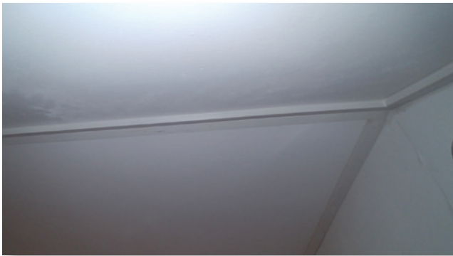
Photo: Close Up Ceiling Trim
